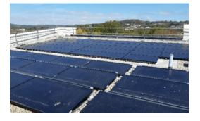
224 photo voltaic panels have been installed, which cover an area half the size of a five-a-side football pitch, on the new office development at Bath Quays South. The development now hosts the largest solar array in Bath and will provide the building with a reliable source of renewable energy.
